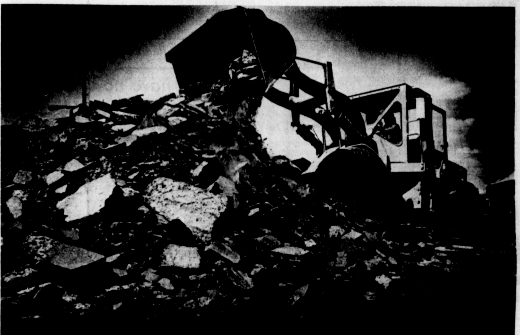
What used to be a several-block stretch of Midkiff Road lies in one large pile with the machinery throwing on more of the crushed street. The city started work Monday on a $1.3 million project to rebuild Midkiff Road from Illinois to Storey streets. The final project will go north to Golf Course Road and include the intersection at Illinois. (Staff Photo by Brian Hendershot)
