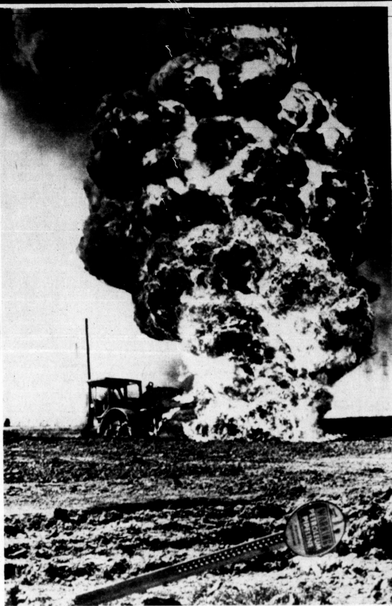
A road grader burns out of control as it sits on top of a liquefied natural gas pipeline that it severed. A six block area was evacuated before the escaping gas burst into flames about forty-five minutes after the accident. (AP Laserphoto)
