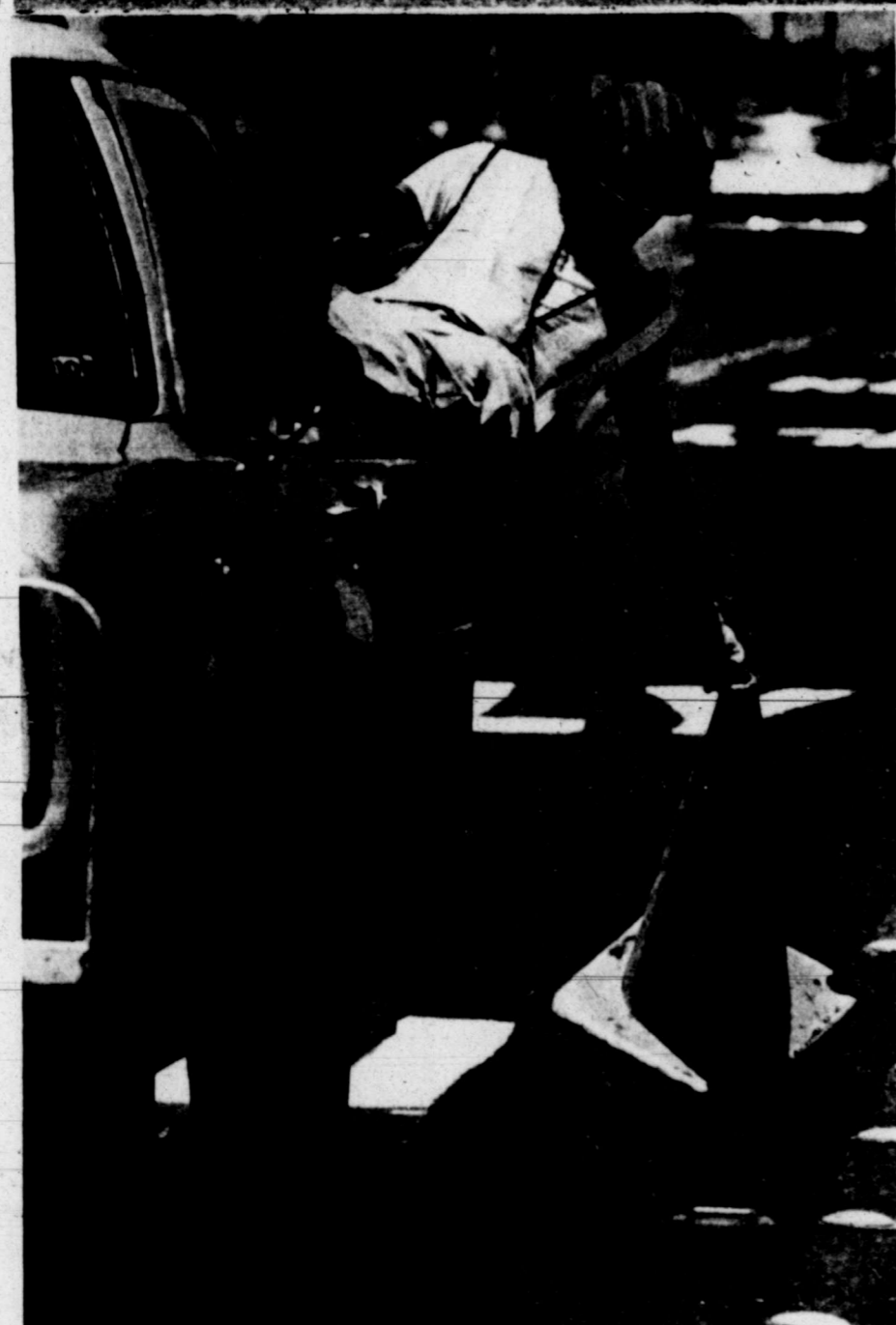
Gerald Conally, left above, of 2300 N. Terrell St., and co-worker Frank Garcia, 1103 W. Kentucky Ave., apply a fresh coat of paint Wednesday afternoon to large-print directions on Big Spring Street. At the left, Garcia snatches up the protective cones after the paint dries, sometimes while in transit to the next job location. Both work for the Texas State Department of Highways and Public Transportation. (Staff Photos by Edward McCain)
