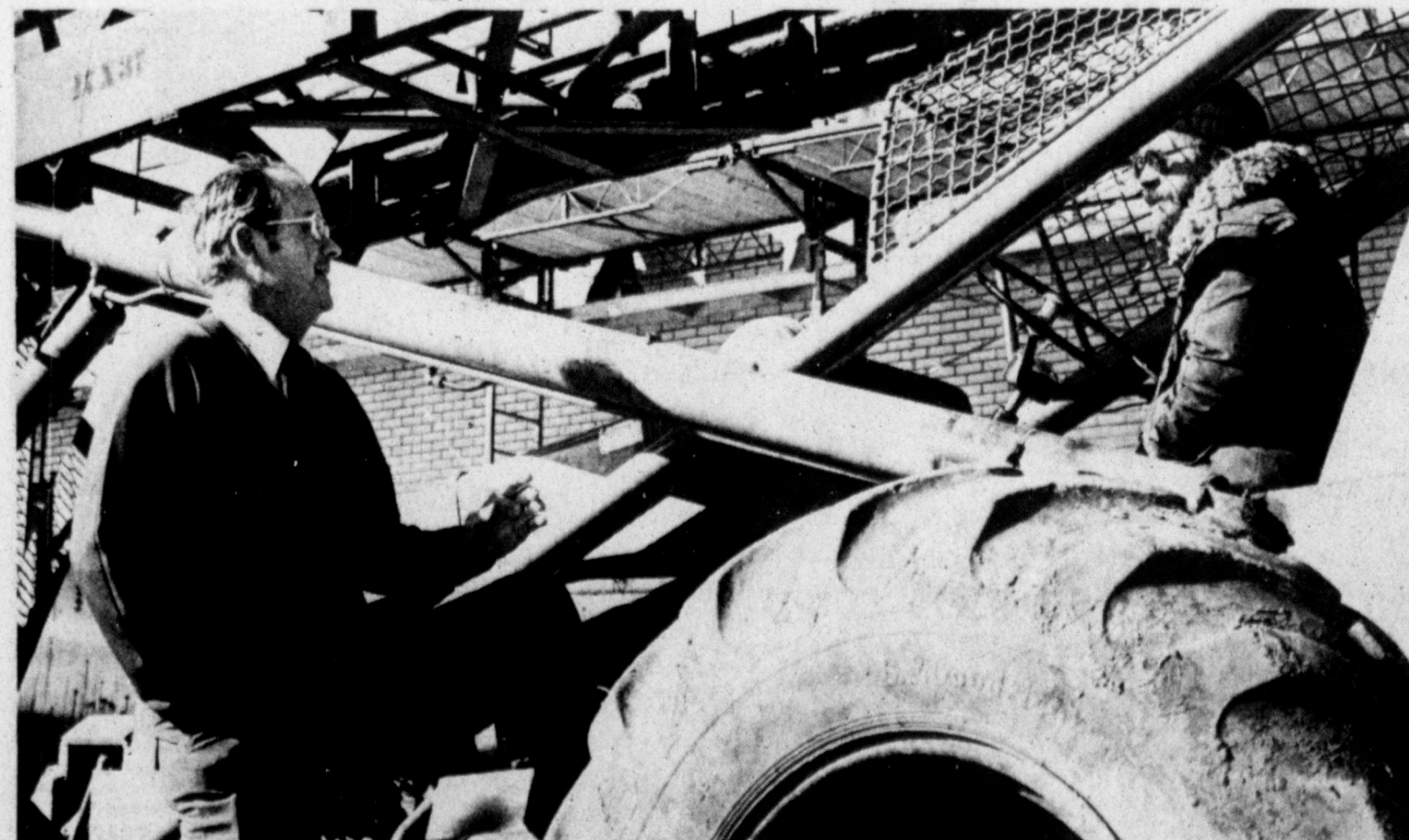
Vitally interested in the future of Midland, Martin Allday, candidate for Mayor of Midland, visits the construction sites of the new mall northwest of Midland.
