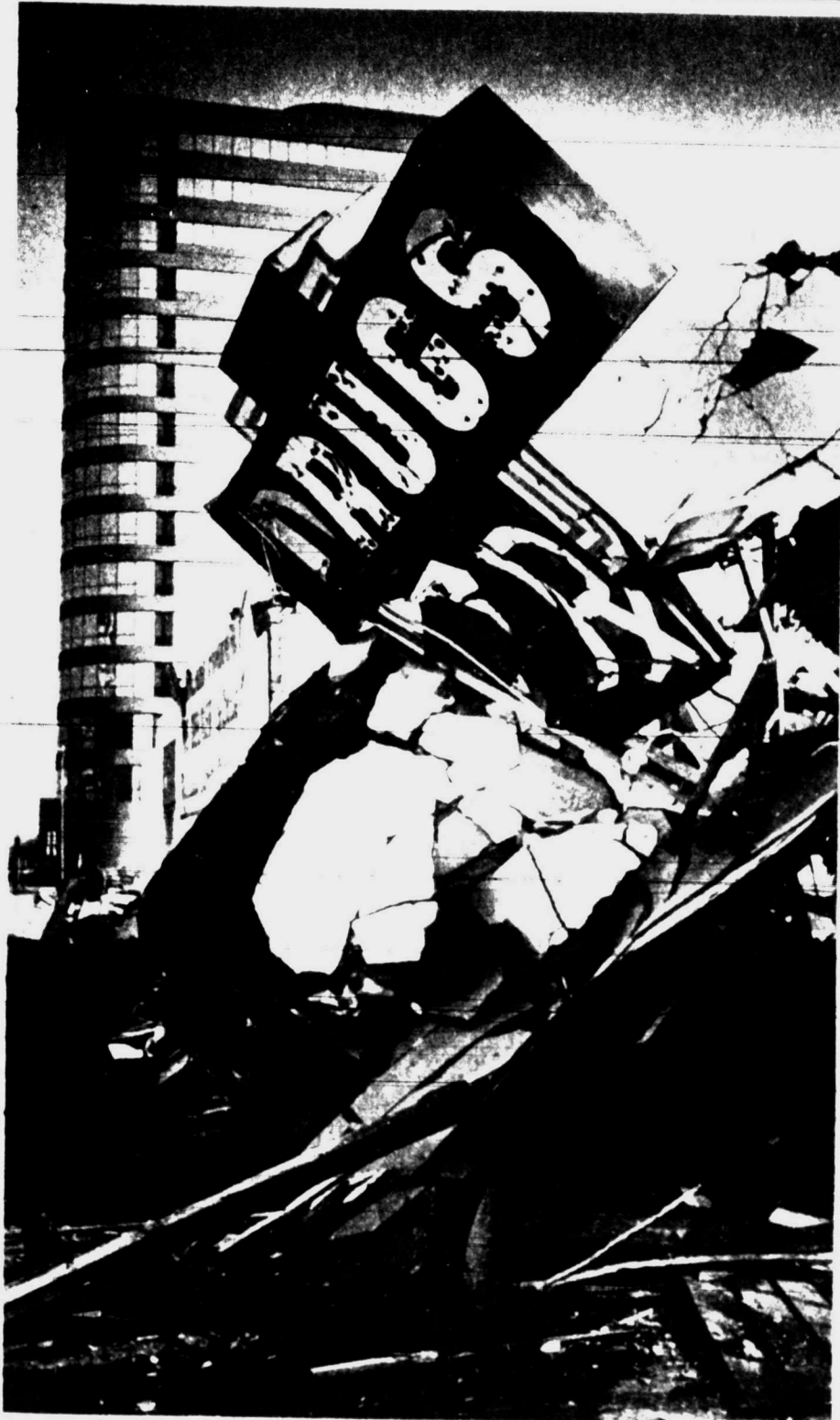
The old Kirkland Drug Store, which in the early 1970s witnessed the scuttling and razing of the old Scharbauer Hotel in downtown Midland, is falling victim to "progress" and to the demolition crew. The old Scharbauer was replaced with another hotel, the Midland Hilton, but only trees, grass and other landscaping for a park will replace the Kirkland. The park, on the same block as the new Midland Center, will complement the center and will also be on ground where once stood the 1930s built post office. (Staff Photo by Brian Hendershot)
