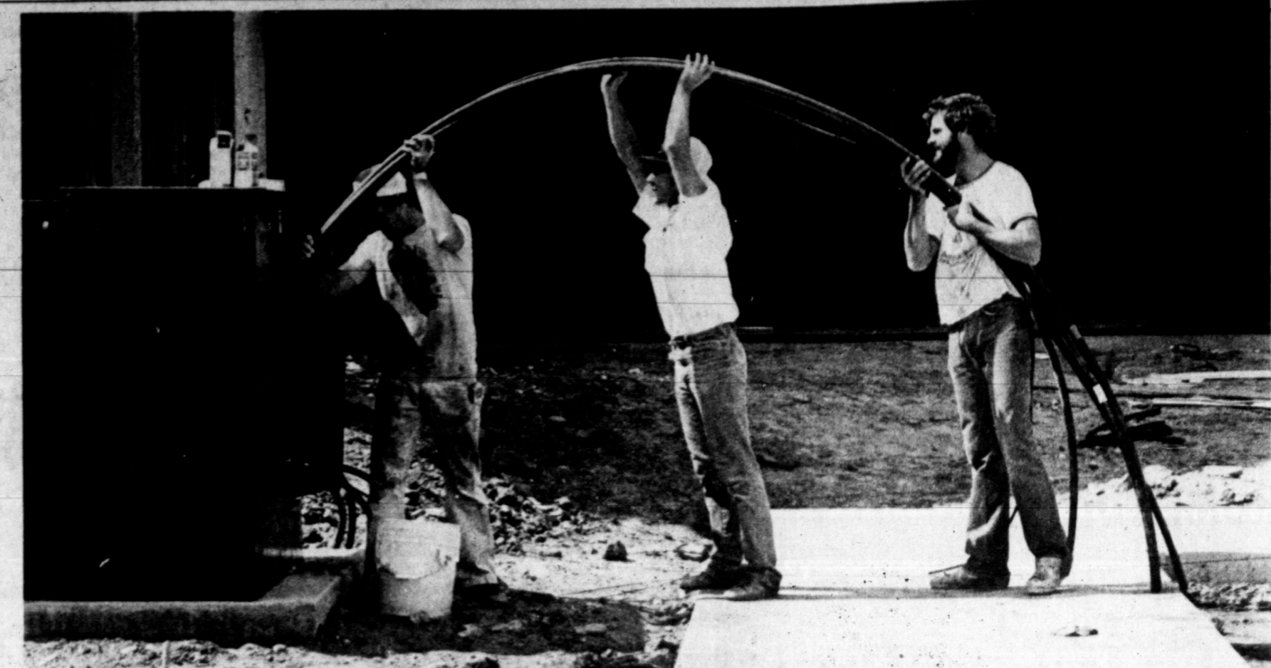
Midwest Electric workers, from left, Jerry O'Brien, Kelly Walker and Larry Belcher push a 135-foot, 600-pound electric cable through underground piping. They were working Thursday afternoon on the new offices at the intersection of Wadley Avenue and A Street. (Staff Photo by Edward McCain)
