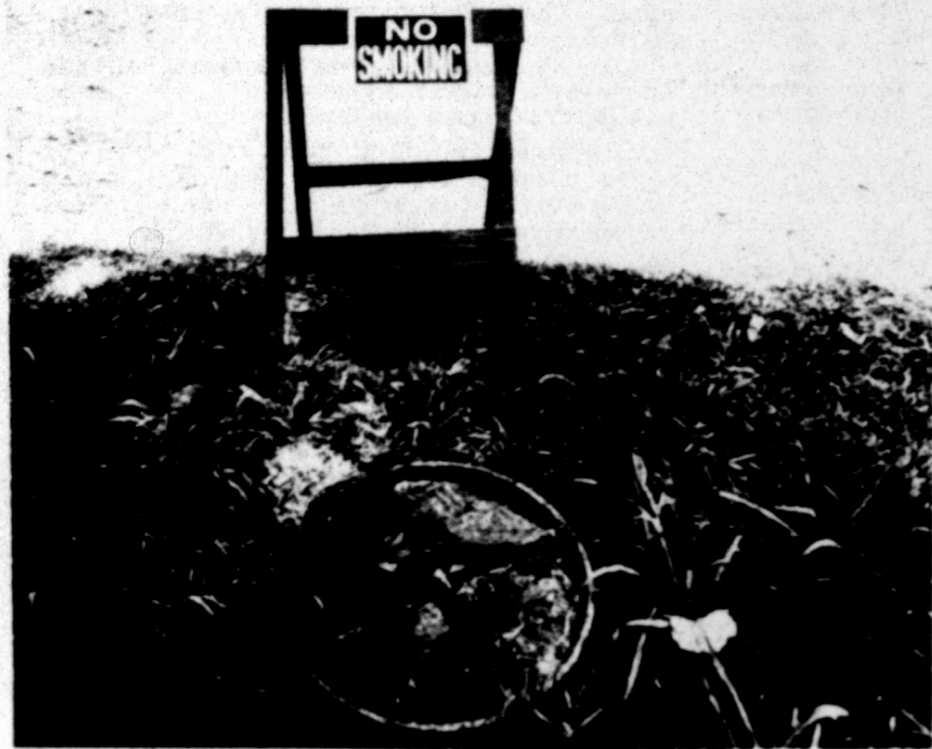
A "no smoking" sign stands over an opened sewer line in Daisetta, warning of leaking gas. The church in the background was closed when dangerous levels of flammable gas were found in it, school buildings and sewer lines. House-to-house checks are under way as the search continues for the source of the gas threatening the East Texas community. (AP Laserphoto)
