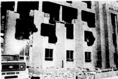
Renovation isn't always neat, even in a hospital. Workmen removed the front wall from the central wing of Midland Memorial Hospital this year to allow the addition of private baths to each room in the wing. The construction is part of a \$10 million project scheduled to be completed by early 1980. (Staff Photo by Mike Kardos)
