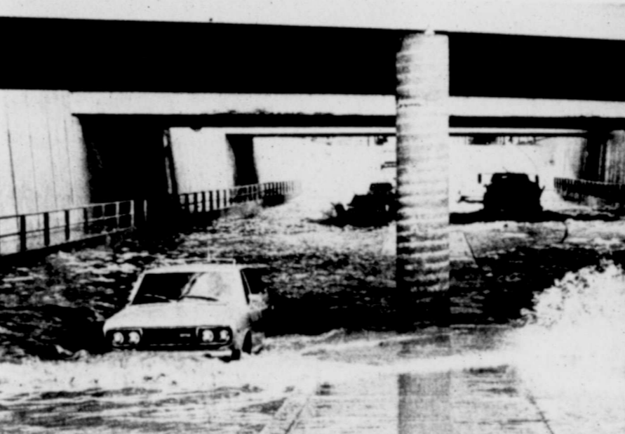
Only a few vehicles made it through the underpass on Big Spring Street at Industrial Avenue Thursday after a storm dumped more than two inches of rain on parts of Midland in slightly more than an hour.
