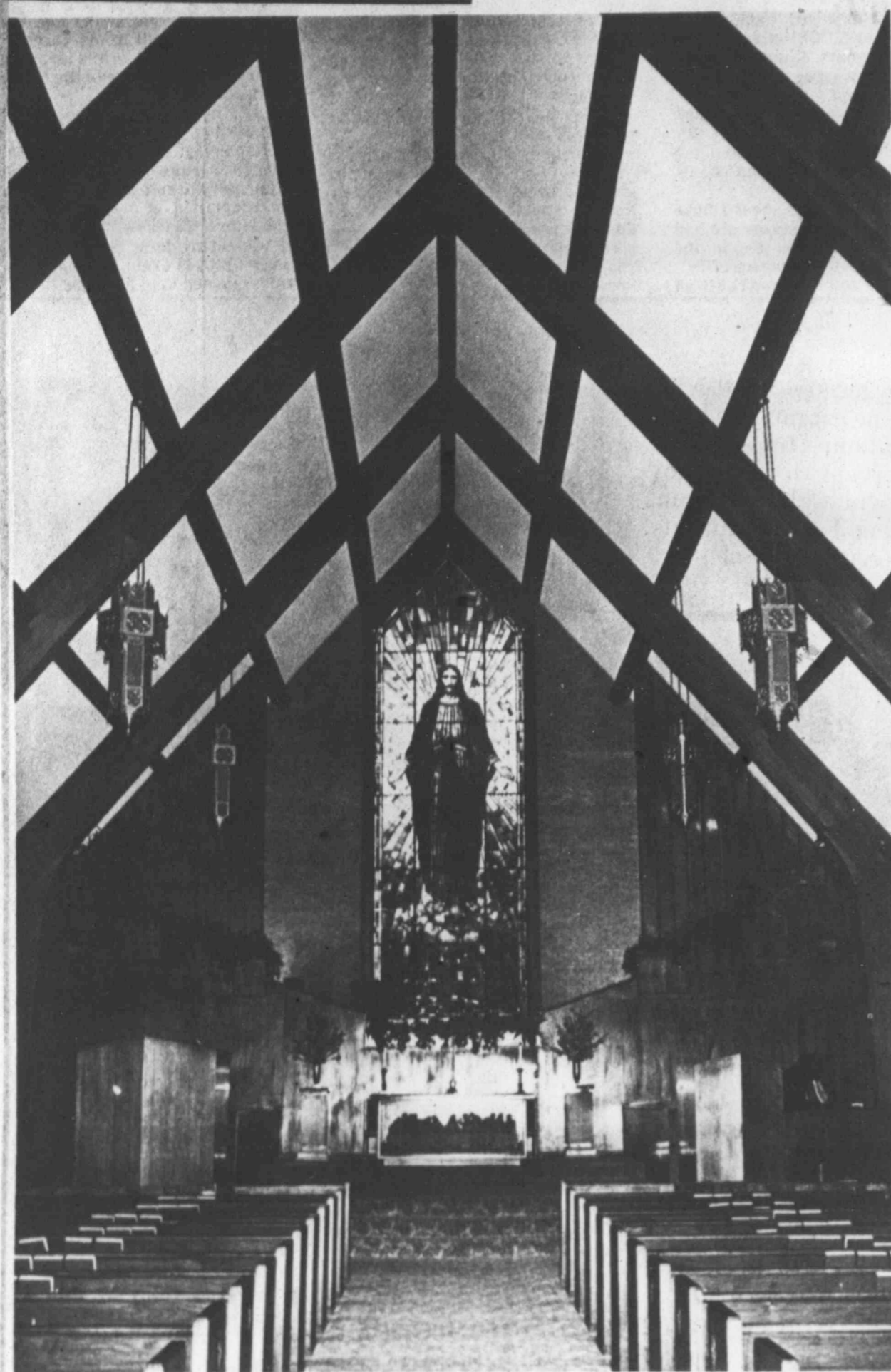
The Sanctuary of the First Christian Church at 1301 West Louisiana Ave. seats about 475 persons on its Canadian walnut pews. Stained glass used in the figure of Christ and in medallions in the side windows was imported from Europe, as was the
