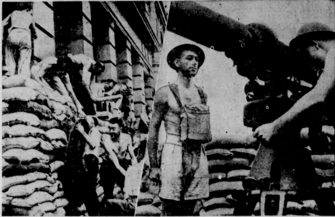
There is no city in Australia that can quietly sit back with the assurance that it will not be bombed by Japs. In the picture at the left, Melbourne city employees are doing their Australia-day task, erecting an ARP sandbag barricade outside of their working premises. Right: Members of the anti-aircraft battery man a height and range-finder at an action station in Darwin, Australia. The men work stripped to their waists.
