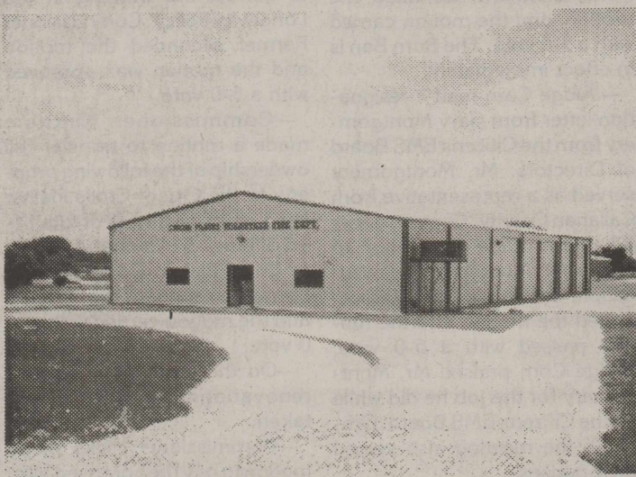
Cross Plains VFD Firehouse
