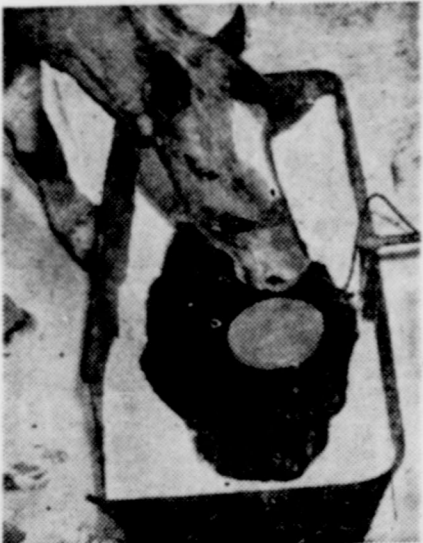
This horse can laugh at Old Man Winter as a result of this floating water heater, an electrical de-icer which assures farm animals a drink despite the cold.
