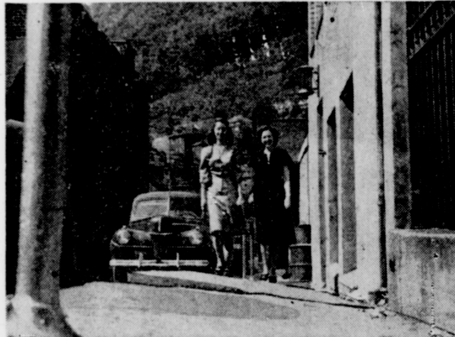
EARTH SHIFTING THREATENS TOWN . . . Two hardy members of the opposite sex, residents of Welch, W. Va., brave a stroll on the buckled streets of the town after sections of the little city started to sag alarmingly because of a mysterious shifting of the earth. Huge cracks appeared in several large buildings, and inhabitants were fearful that their homes would be destroyed.
