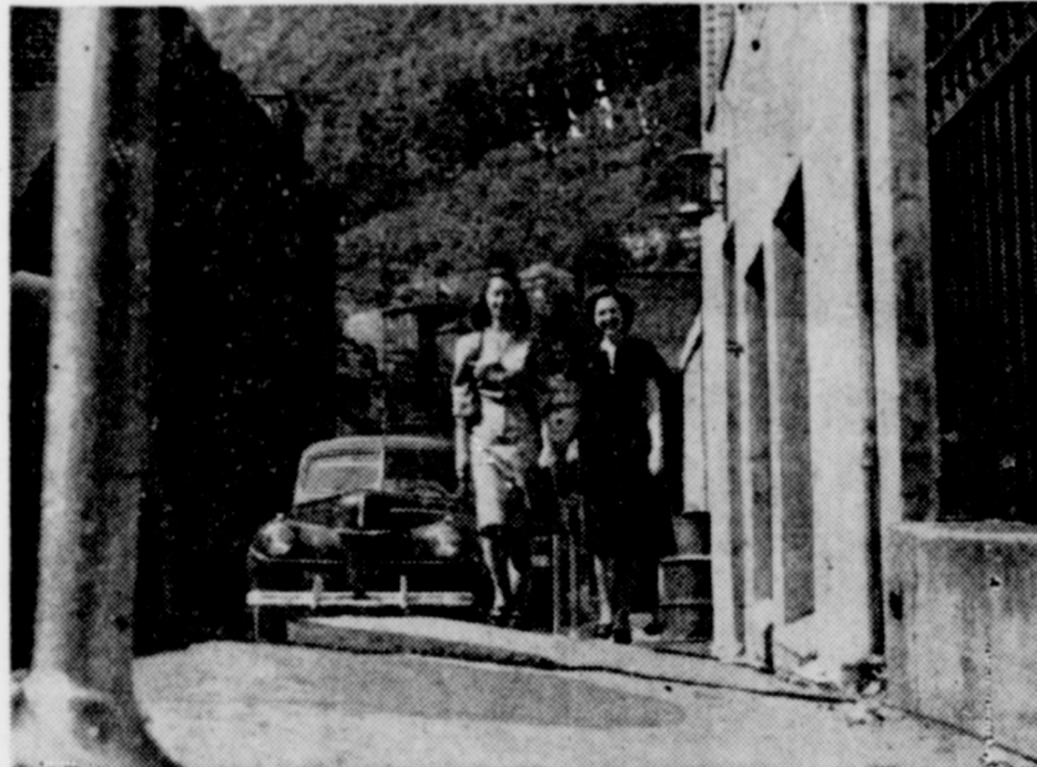
EARTH SHIFTING THREATENS TOWN . . . Two hardy members of the opposite sex, residents of Welch, W. Va., brave a stroll on the buckled streets of the town after sections of the little city started to sag alarmingly because of a mysterious shifting of the earth. Huge cracks appeared in several large buildings, and inhabitants were fearful that their homes would be destroyed.
