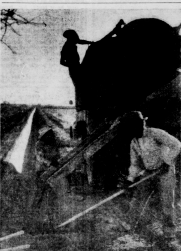
WORKMEN POUR CONCRETE in completion of an irrigation ditch for the tract of ground that is being bench levelled on the Bowman farm. (Advocate Photo)
