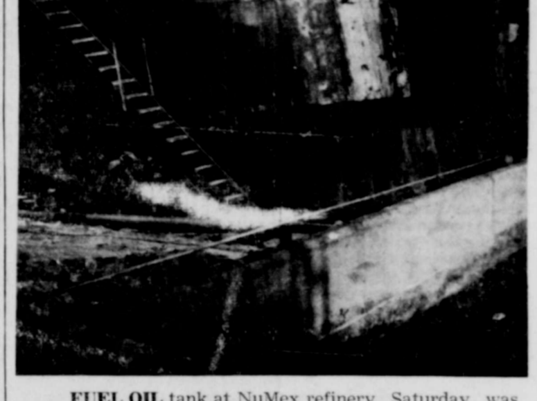
FUEL OIL tank at NuMex refinery Saturday was crumpled and shaken from its foundation by explosion, which workmen theorized happened when hot fuel oil touched off blast. Tank was shaken from its foundation. There were no injuries reported. Damage has not yet been estimated. (Advocate Photo)
