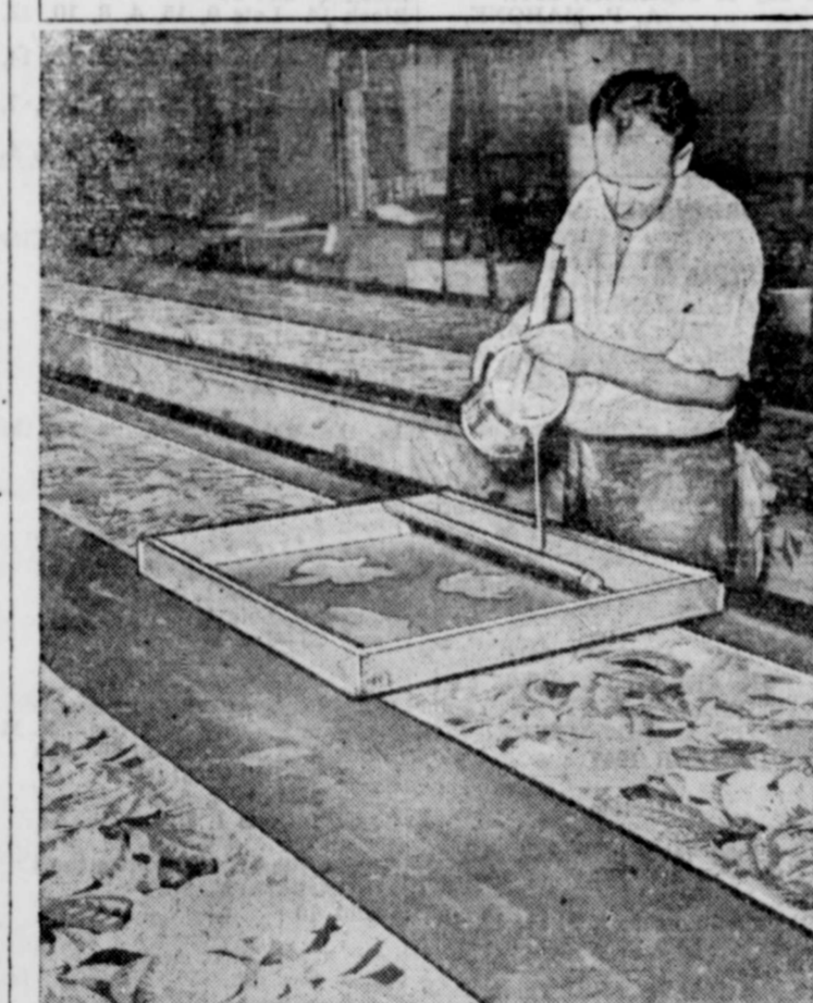
Frank Wilson, of Gibson, Long Island, is about to hand-screen another color onto wallpaper at Inez Groom, Inc., New York City. Both paint and paper require fats and oils in their manufacture.
