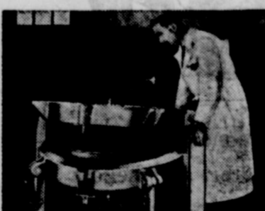
Curing Firestone New-Tread in Old Tire
