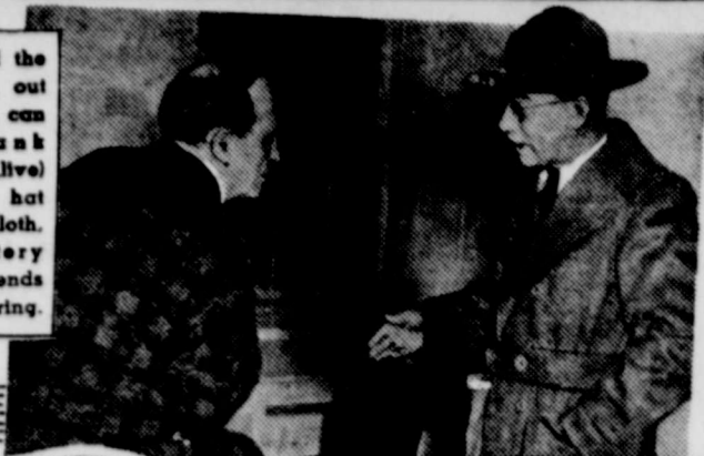
MARTIAL LAW established by Oklahoma over $20,000,000 State-Federal Grand River Dam. as Major H. B. Parria, Oklahoma National Guard, confers with Construction Superintendent Towne.
