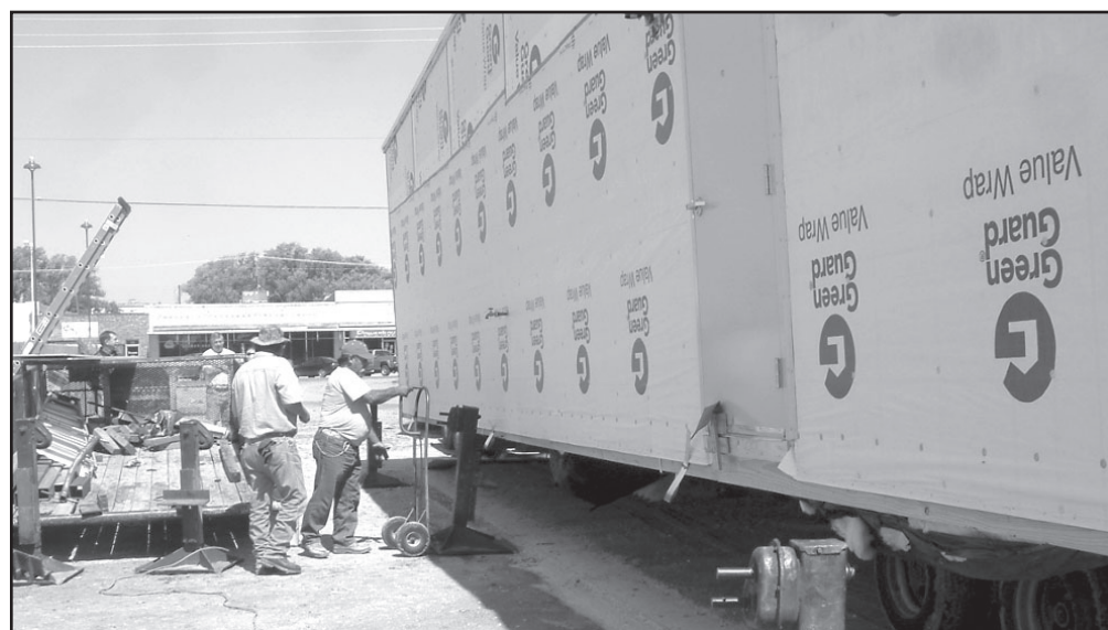
Workers prepare to set the first police department module in place Tuesday.
