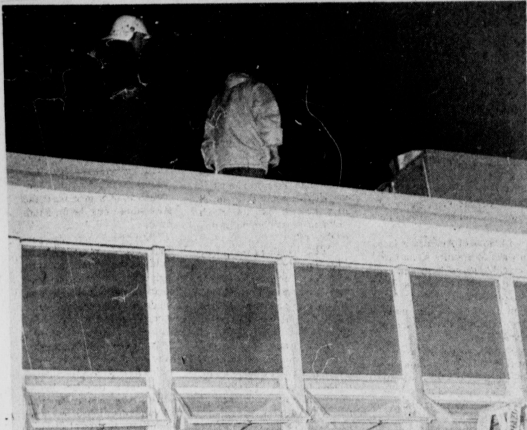
CHECKING FIRE... Cold firemen were on top of DeShazo School early Saturday night checking the results of a fire which damaged the east wing of the school. The fire which started in the heating unit shown, apparently blazed up, alerting a nearby homeowner, Lester Elmore, who first reported the fire. Edwin Cox drove upon the blazing unit, and also notified authorities. Apparently no severe damage resulted, although students are attending class in a 'cool' building.
