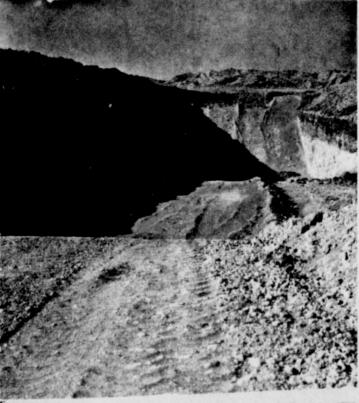
DAILY PIT . . . . This pit is one of five at the sanitary landfill. It is where daily gargabe is dumped and buried each day. The picture shows the pit after several weeks of garbage have been dumped in the pit and buried each day. The garbage is first compacted then covered with six inches of soil.
