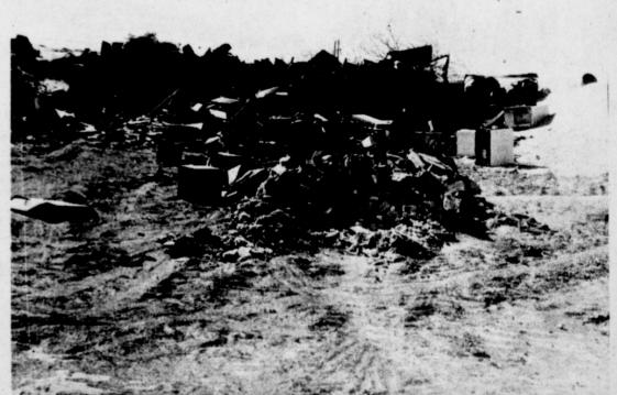
METAL PIT . . . . . This pit is the one that is used for metal, old stoves, refrigerators, tin and wire. The trash is compacted and buried when enough accumulates. The accumulation shown here is about a month's worth of garbage. It will be compacted and covered with six inches of soil like
