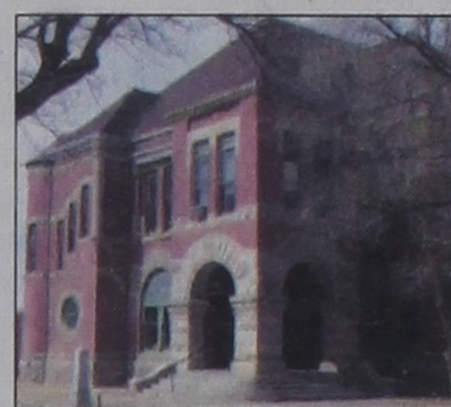
The Donley County Courthouse before restoration.
