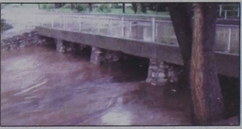
A view of the Kearney Street bridge at Fifth Street.
