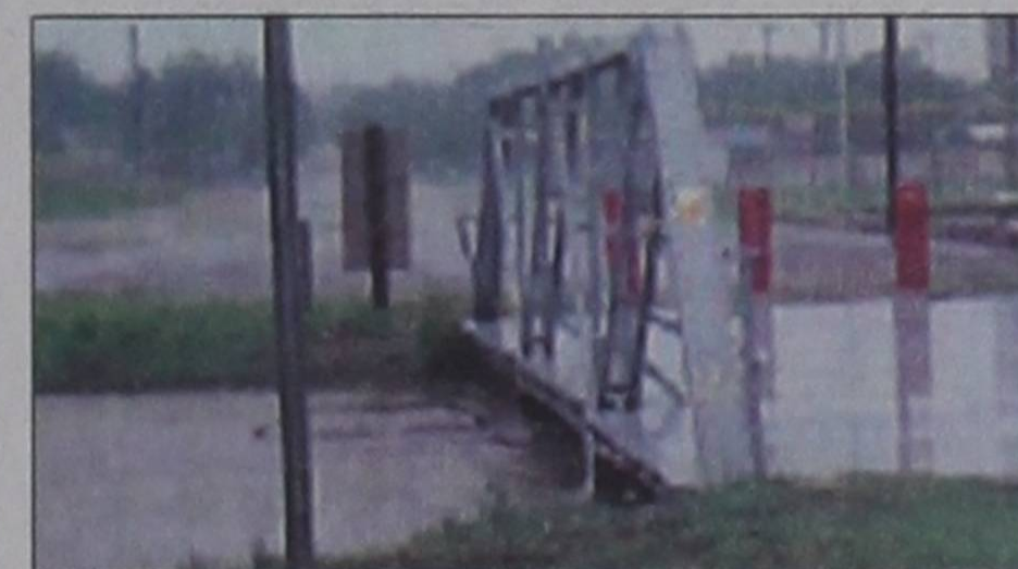
Water flowing under the Seventh Street truss bridge at City Park.
