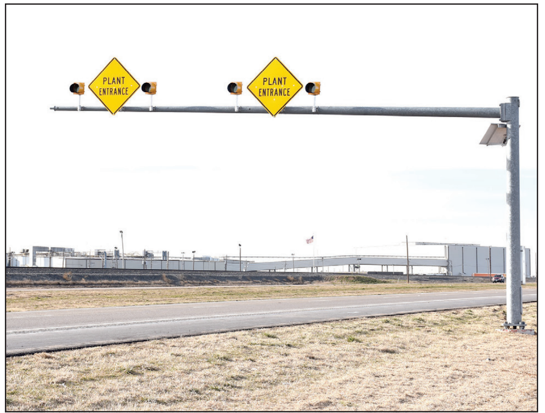
Flashing lights and rumble strips have been installed on Highway 60 with the intent to make the entrance to the Friona Cargill Plant more safe. The company is looking to obtain funding for an overpass to be located west of its facility.
