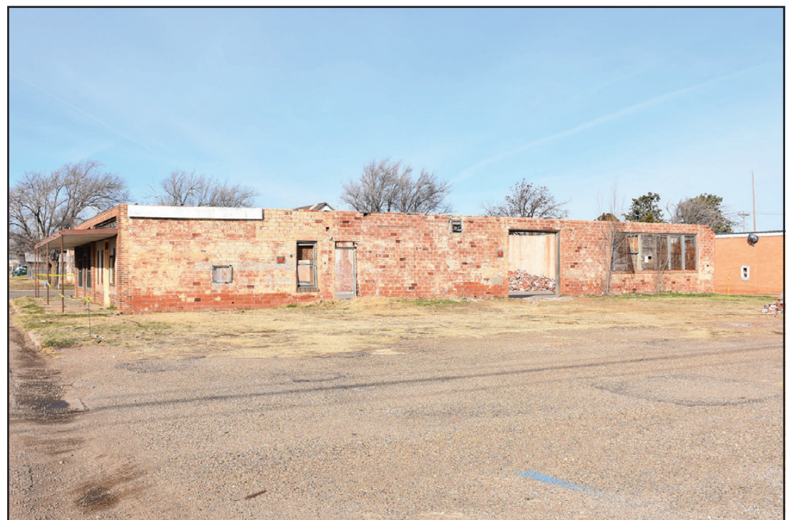
Work is being done on the old movie theater on 6th Street. A new roof will be installed and plans are for the building to be used as a warehouse.
