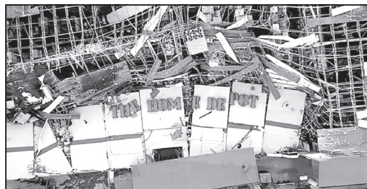
Aerial image shot by a drone shows a Home Depot store in Dallas, Texas, that was obliterated after a destructive nocturnal tornado ripped through the area on Sunday, October 20, 2019. (SevereStudios / John Humphress)
