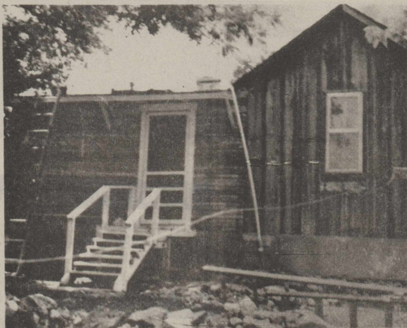
The Sonora Volunteer Fire Department's Christmas in April Project. Before
