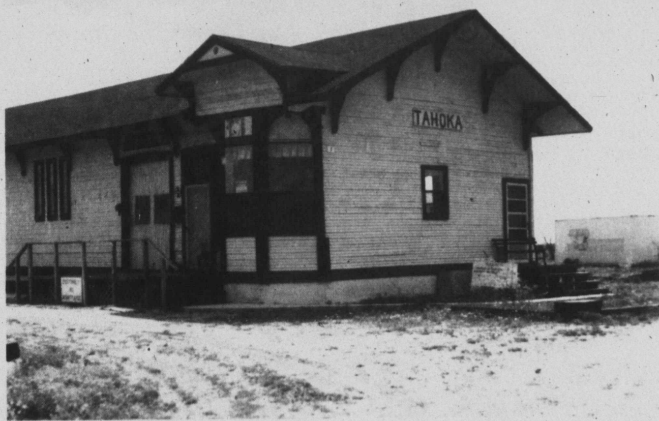
OLD TAHOKA DEPOT REMODELED - The old Santa Fe depot at Tahoka, built in 1910, is now remodeled into a country home, located between Winters and Wingate. The Lynn County News ran an article about the depot two weeks ago, and Mr. and Mrs. Robert Draper of Tahoka were travelling in that area recently and took this photograph. The remodeled depot is owned by Rita Stephenson, whose family uses the home for family gatherings.
