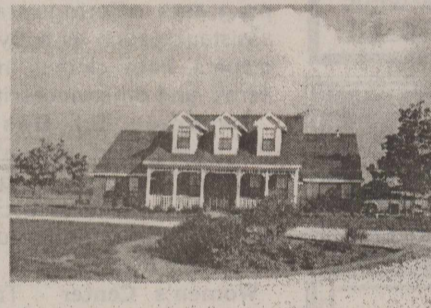
Beautiful country home, quality construction spacious open living area with rock fireplace, entertainment center and gorgeous master bedroom. 3BR, 2B. 40 X 60 all metal barn. Extra ranch home west side of property.
