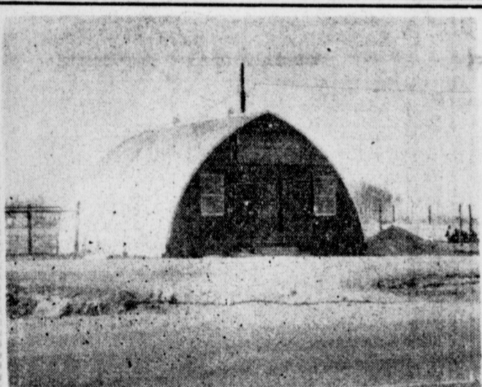
New Office and Pipe Yard Located North of Muleshoe
