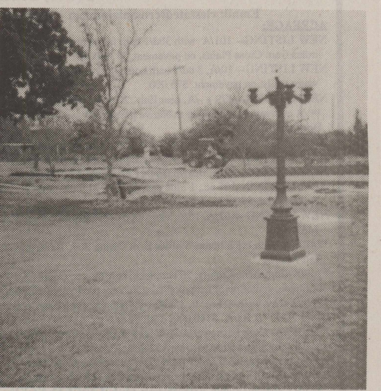
NEW PARK BESIDE CITY HALL—The cement work on the fountain and gazebo have been completed. A paved stone wall adds charm to scenery, along with the street lamps. Watch to see what is added each week.
