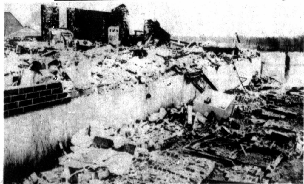
THE CHARRED REMAINS of the Straughan's Wayside Inn nursing home following a fire that killed 25 persons. Officials now say all the residents could have been saved. See page 6 for details.
