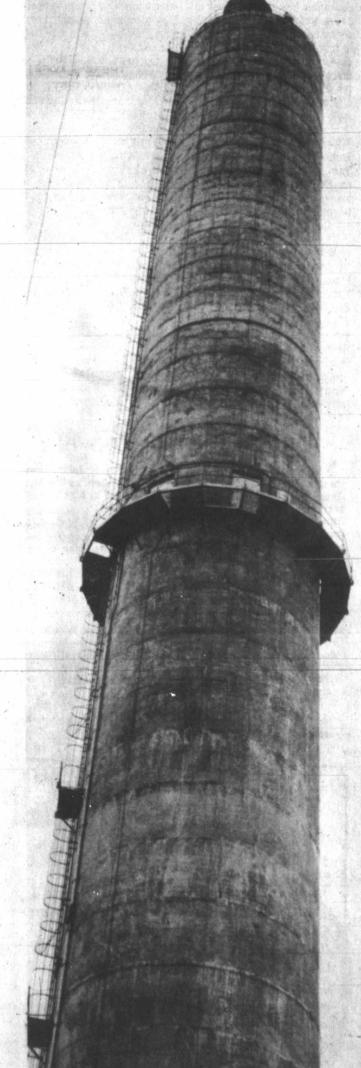
THE STACK, which dispenses vent combustion gases from the boilers at the properly regulated
