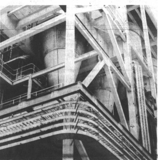
FROM THE BINS the crushed coal is conveyed to the 7 - ft. high boiler structure and into the steam generator storage silos, which are vented to the atmosphere through wet scrubbers.
