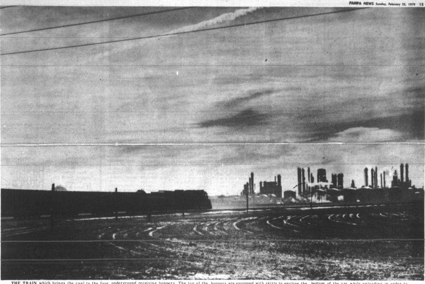
THE TRAIN which brings the coal to the four underground receiving hoppers. The top of the hoppers are equipped with skirts to enclose the bottom of the car while unloading in order to contain the associated air - born dust
