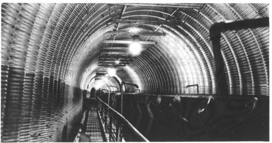
INSIDE THE CONVEYOR which transports the coal from the four underground receiving hoppers to the stacker. From here the coal is conveyed to the crusher where it is reduced to a size
