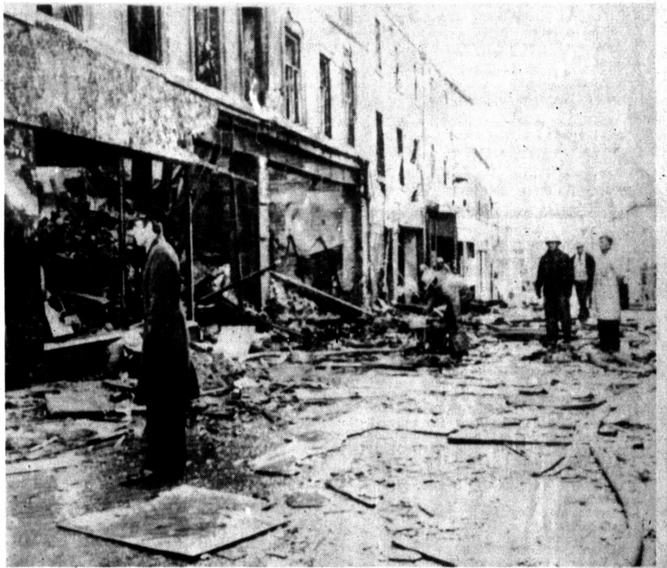
BLAST DEBRIS is viewed by members of the police and fire services Friday morning after a huge Irish Republican Army car bomb exploded Thursday night on Scotch Street in the center of Armagh.
