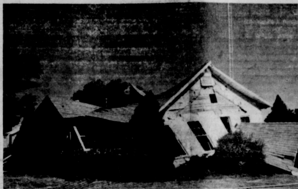
THIS HOUSE, just vacated by former Station superintendent Charles E. Fisher, blew up at the Experiment Station last week while it was being fumigated. Paul C. Marion, Fisher's successor at the Experiment Station, along with Ed Webb, city employee who runs the fogging machine, had just finished spraying when the blast occurred. Butane trapped under the house is believed to have caused the blast. Marion was to have moved into the house the day after it blew up. —Photo By MORGAN
