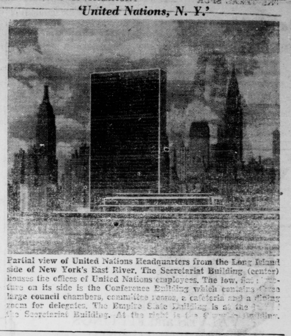
Partial view of United Nations Headquarters from the Long Island side of New York's East River. The Secretariat Building (center) houses the offices of United Nations employees. The low, flat building on its side is the Conference Building which contains the large council chambers, committee rooms, a cafeteria and a dining room for delegates. The Empire State Building is at the right is the Secretariat Building. At the right is the Secretariat Building.
