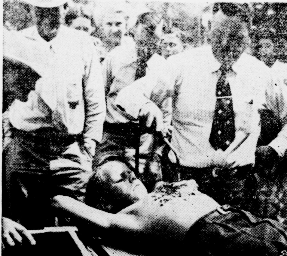
WICHITA, KANS. — Don't be alarmed . . . this is only an educational feature typical of southwest state fair demonstrations by a manufacturer of home and building insulation. Amazed spectators watch as a company representative subjects a few inches of Insul-Wool insulation on the youngster's chest to the steel-melting heat of an acetylene torch. No fire and no harm to the youngster.
