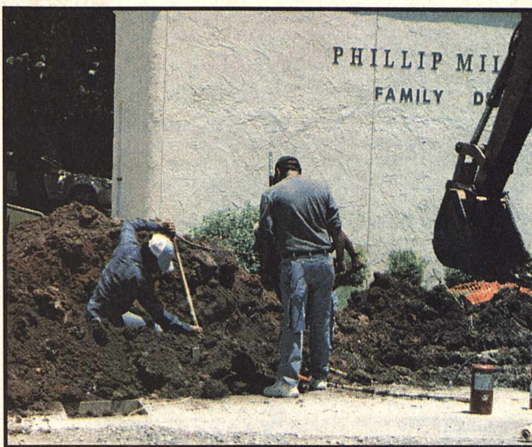
Crews scramble to repair broken gas line
