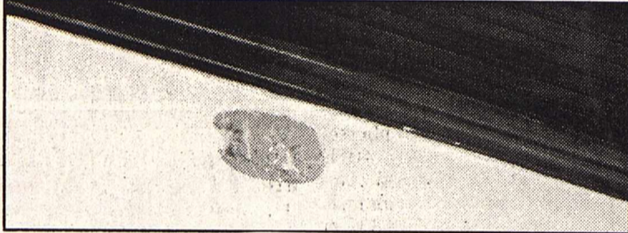
(Above) An architect searches under years of paint for original stenciling on the Sutton County Courthouse walls. (Below) Original stenciling is found under coats of paint in the front entrance way.
