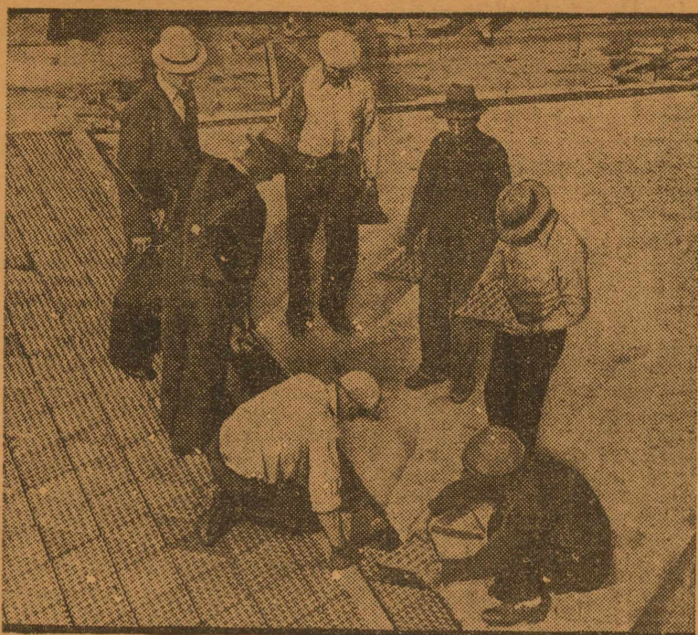
Cast iron paving made its debut in the United States when a thirty-foot strip was laid at the University of Minnesota in Minneapolis for a test to determine its possibilities on a national scale.
