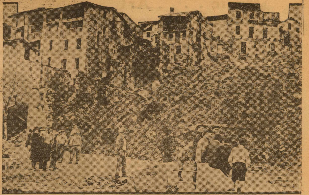
A scene in the town of Roquebillieres, not far from Nice, France, just after the town had been evacuated as a heavy landslide caused by torrential rains covered many of the homes and crushed others in its path.
