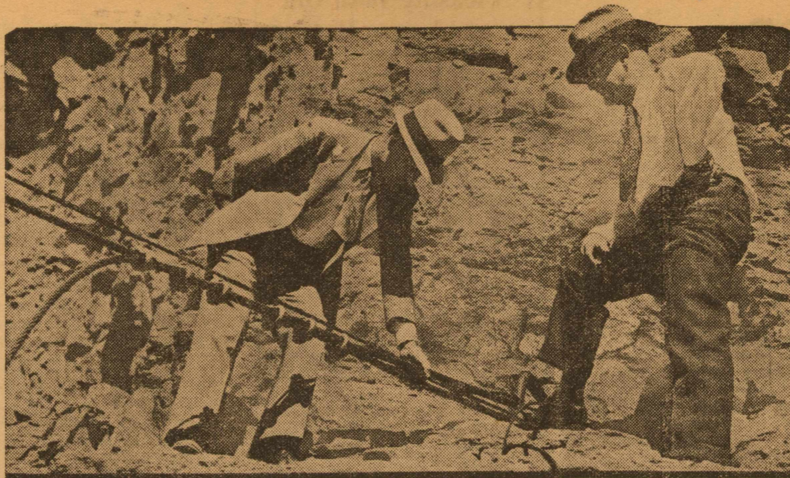
Maj. F. I. Pomeroy of the Arizona National Guard announced that Arizona's rights had been encroached upon through the anchoring of several cables in Arizona territory in the sensational state squabble over construction of the Parker diversion dam by the metropolitan water district of southern California.
