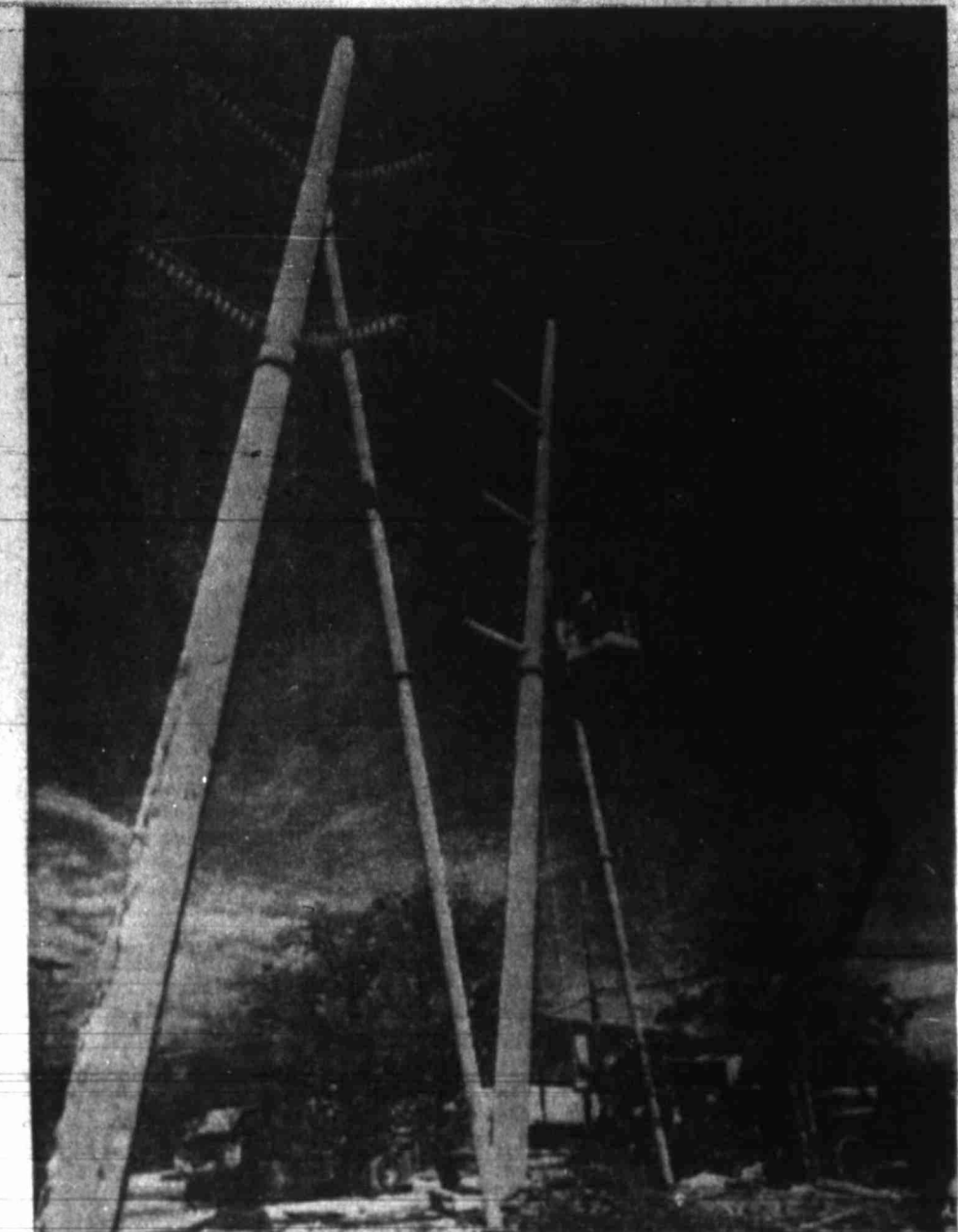
ANGLED — An unusual pattern was formed by high-tension power lines being erected in Fort Worth recently. The lines were put in place by a cherry-picker. (AP Wirephoto.)
