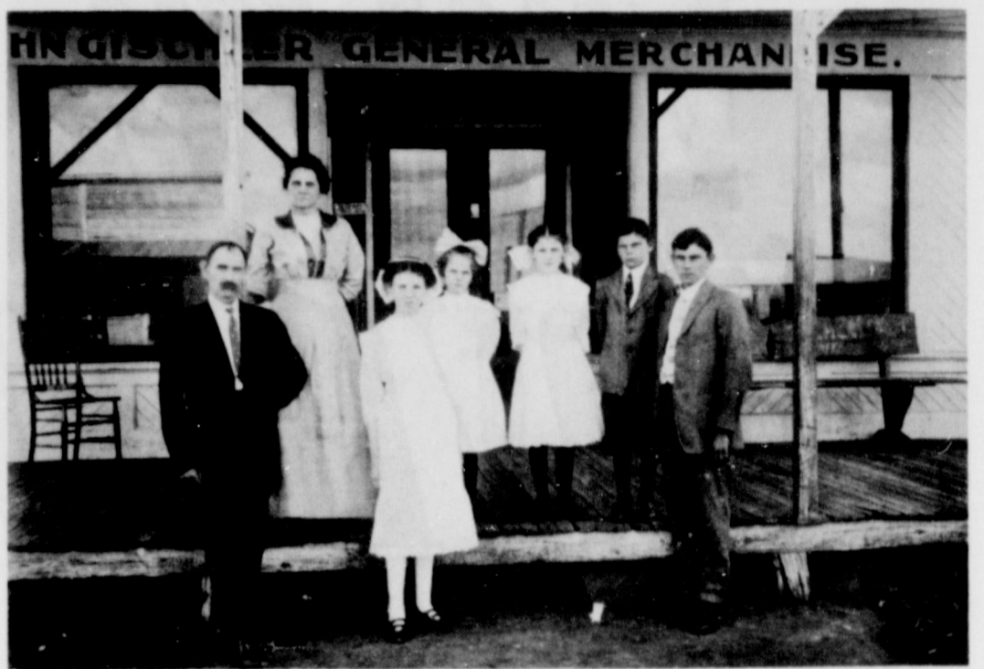
ORIGINAL BUILDING. . . The above building, which was located at Sixth and Main Streets, where Friona Credit Union is located today, was the first location of Friona State Bank, which opened its doors as First State Bank on June 1, 1908. The above shot, taken a few years later when John Gischler had a general merchandise store at the location, shows the Gischler family. Left to right are Mr. and Mrs. John Gischler, Luella (Mrs. Carl Maurer), Constance (Mrs. Lawrence Walker), Viola (Mrs. George Treider), Ruben and Elwin Gischler.
