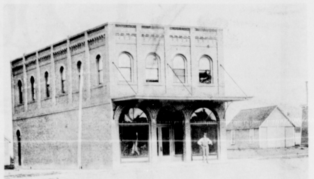
OLD LOCATION. . . The location used by Friona State Bank for some 40 years, at Fifth and Main, is shown shortly after it was completed, sometime in 1910. The building was used in recent years as the Masonic Hall, and now is owned by the Calvary Baptist Church for its mission.
