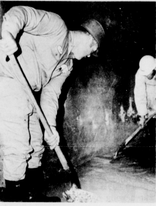
CLEANING WORK. . . This series of pictures shows work being done by City of Friona employees this week in cleaning out sand which collects yearly in a city water storage tank. The ground storage tank at Sixth and Grand, after being drained, was cleaned of approximately two yards of sand. City officials said this was about half the usual amount cleaned from the tank. Working inside the tank are Albert Wolfington and Don Powell. Shown on top of the tank are P.C. Aragon and Lewis Murietta.
