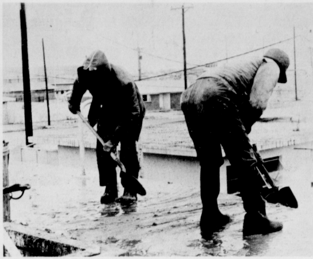
CLEANING WORK. . . This series of pictures shows work being done by City of Friona employees this week in cleaning out sand which collects yearly in a city water storage tank. The ground storage tank at Sixth and Grand, after being drained, was cleaned of approximately two yards of sand. City officials said this was about half the usual amount cleaned from the tank. Working inside the tank are Albert Wolfington and Don Powell. Shown on top of the tank are P.C. Aragon and Lewis Murietta.
