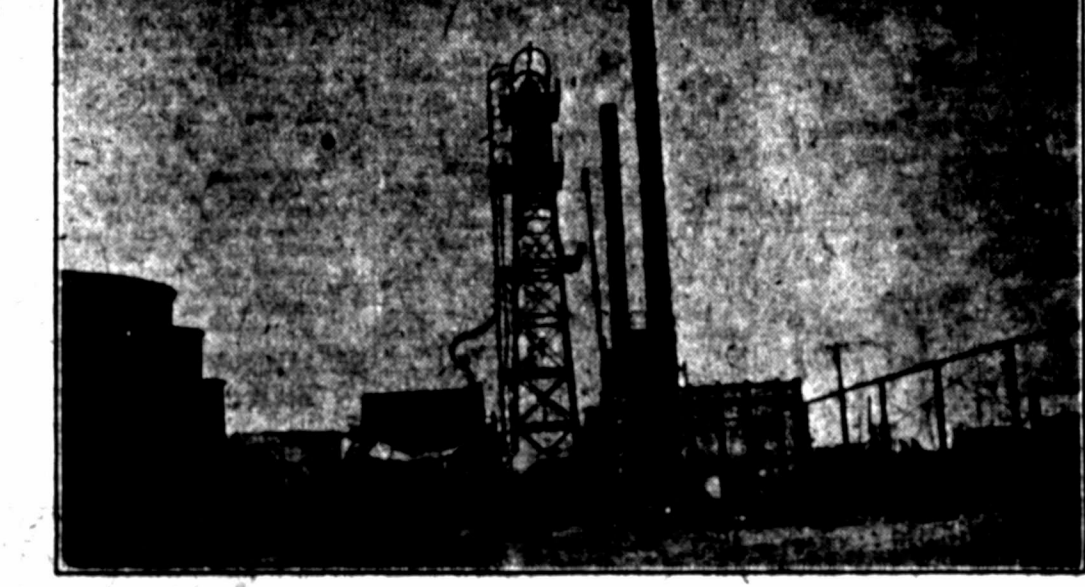
The Panhandle Refining Co.'s unit which will be in operation before the end of August.
