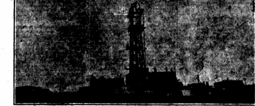
The American Refining Company's plant was the last to be started, but is making steady progress.
