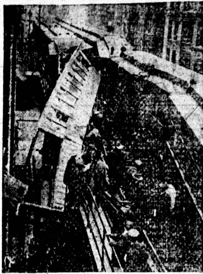
A score of persons were injured, many seriously, when a southbound express train of the Ninth Avenue N. Y. elevated line crashed into a southbound local of the same line, hitting the latter to the street. Photo shows the rescue party at work.
