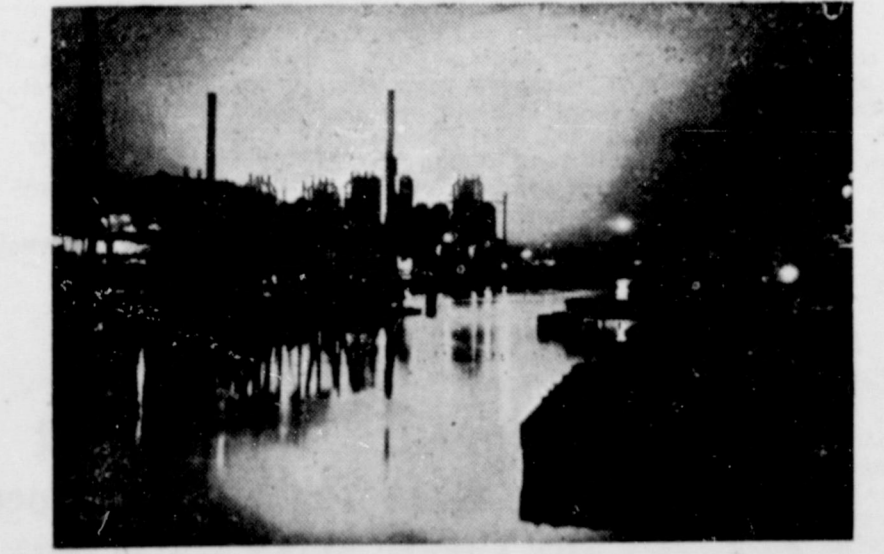
The vast Carnegie-Illinois Steel corporation in Chicago makes an impressive view at night as the glare from converters and blast furnaces cast a ruddy glow in the sky and silver the quiet river. Great plants like this throughout the nation are working at almost capacity production on 24-hour shifts to meet defense needs.
