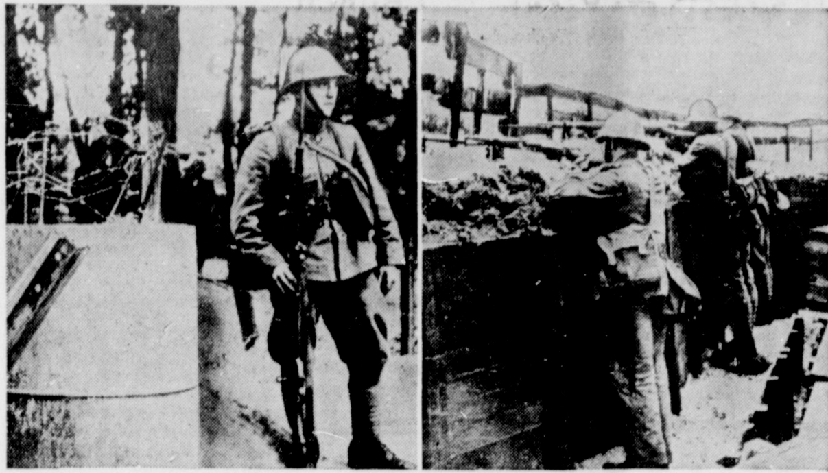
"Somewhere in Holland too close to Germany" is the only locality identification given for this show of Dutch preparedness on the German border. Left: A steel-helmeted sentry stands guard before the entrance to one of the new border fortresses. The concrete stub is a "tank stopper," garnished with steel rails and a bouquet of barbed wire. Right: Soldiers of the Netherlands' regular army stand guard in a trench along the German border. Such scenes are plentiful along the entire frontier.
