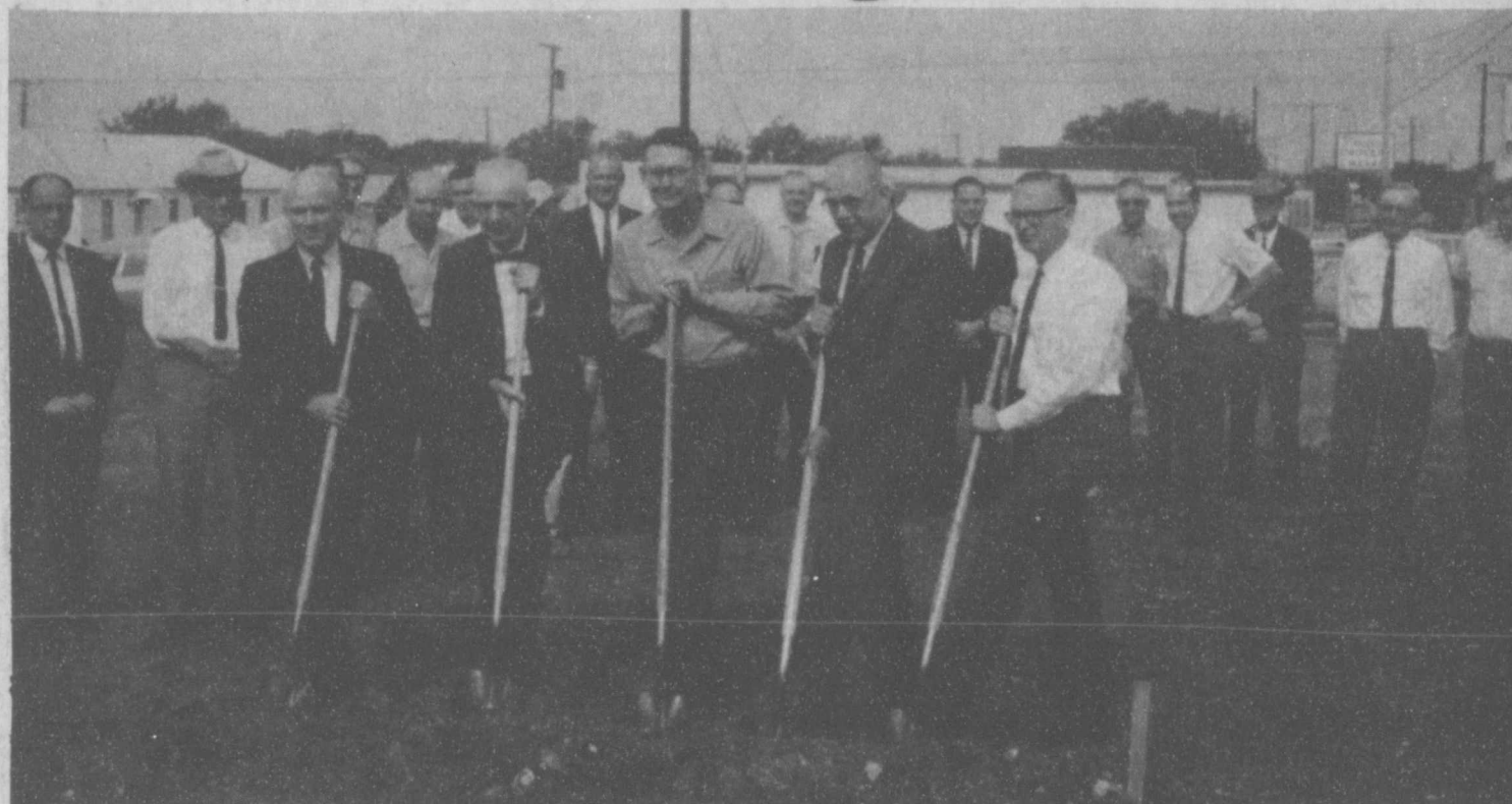
Masons break ground at the site of their new Lodge 197 building, Thursday, May 9th at 10:00 a.m. The Lodge has been working toward this event for three years. Pictured with the shovels, are, left to right: H.K. Jackson, Jr., W.D. Cooper, Erie Powell, (Grand Master), H.K. Jackson, Sr., and Jack Straw (Deputy District Grand Master). The Lodge will hold a cornerstone laying ceremony in a month with Grand Lodge of Texas Grand Master, J.W. Chandler, present.
