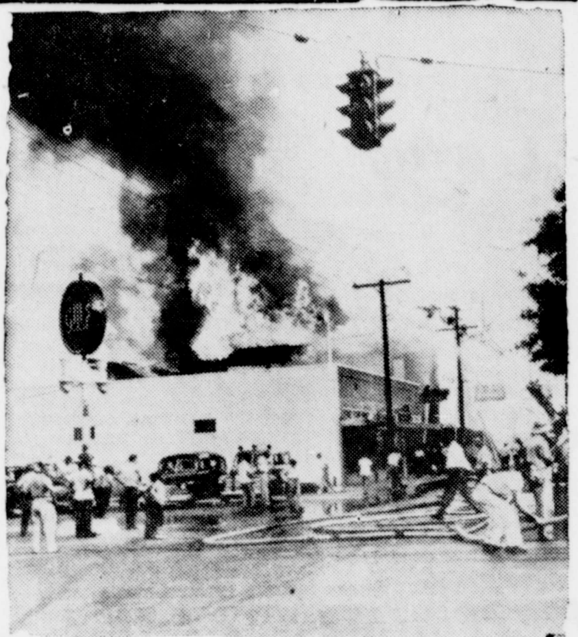
ORANGE BUSINESS BUILDING BURNS
